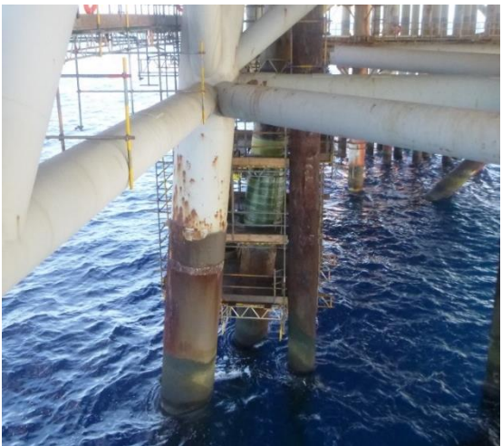
Caissons designed for 100 and 1000 year wave loading
