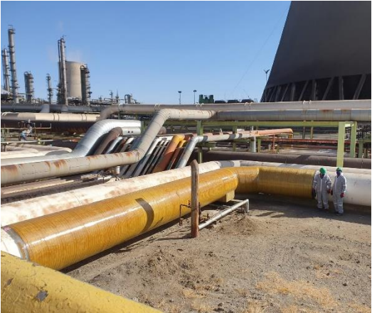
Large OD Cooling Water Lines
