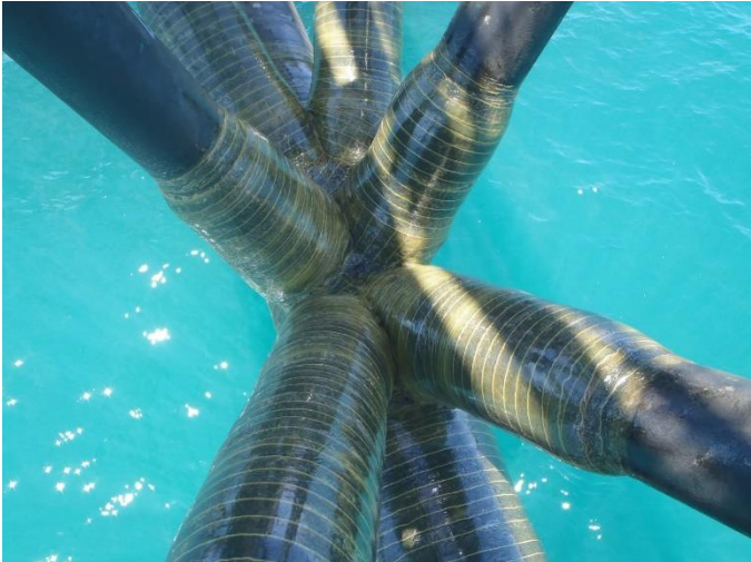
Structural Repair to Jetty
