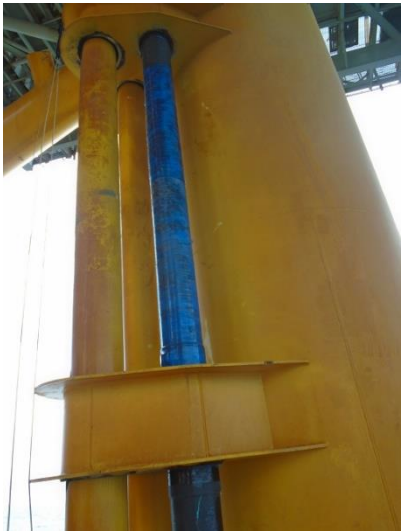
Caissons designed for 100 and 1000 year wave loading
